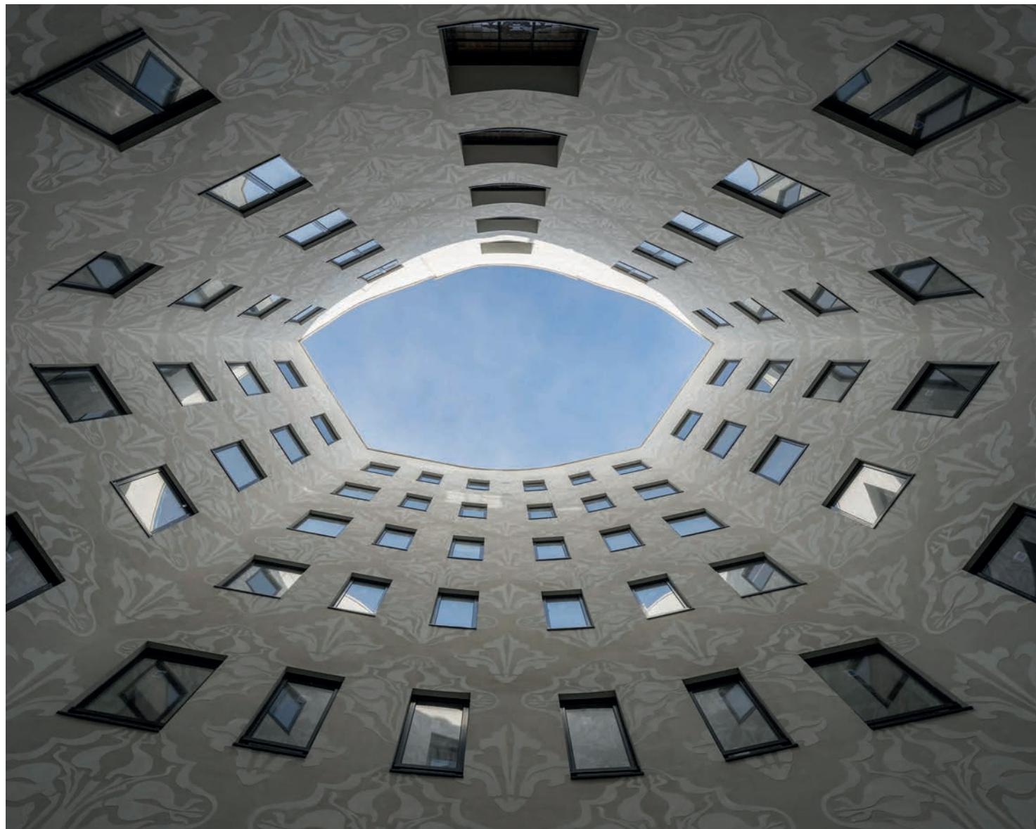
PIEL TÉRMICA INTERIOR CON SISTEMA SATE BAUMIT STARSYSTEM (EPS 8CM, NANOPORTOP FINE, COLORES LIFE 0016, 0019). INTERIOR THERMAL SKIN WITH SATE BAUMIT STARSYSTEM SYSTEM (EPS 8CM, NANOPORTOP FINE, LIFE COLORS 0016, 0019).
